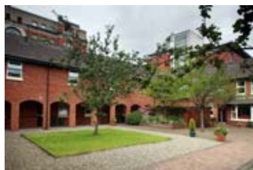
Refurbishment of Chapelfields Fold, Belfast.
